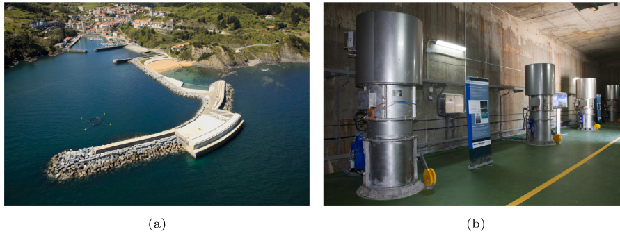
Fig. 1. (a) Exterior view of the Mutriku Wave Power Plant; (b) Interior view showcasing one of its turbines.
